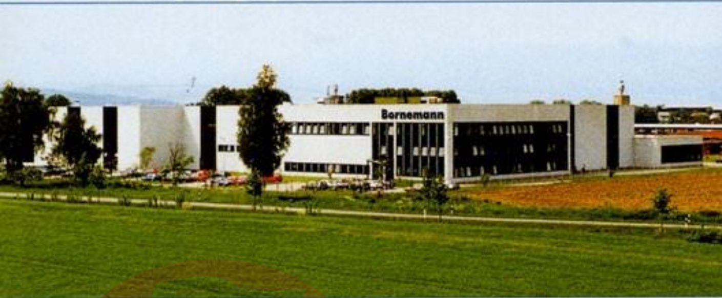
Headquarter of Joh. Heinr. Bornemann GmbH in Northern Germany.
